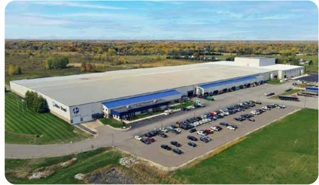
Pictured above, the Alro Steel facility in Pottsville, Michigan
