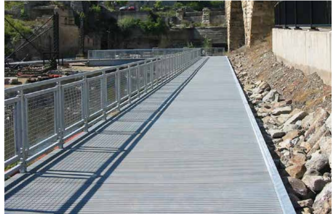
Mill Ruins Park in downtown Minneapolis, Minnesota utilized DURAGRID® T-1800 1" for new pedestrian walkways in the beautiful historical district.
