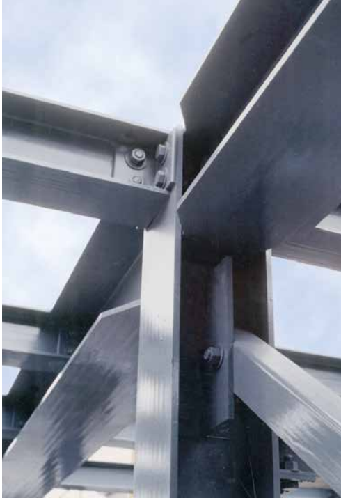
Bolts and adhesives are used for efficient connections in EXTREN® structures.
