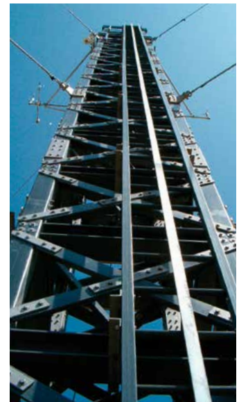
A 62' (19.5m) tall weather tower at Vandenberg Air Force Base near Santa Barbara, California is composed of EXTREN® structural shapes, ladders and DURADEK® pultruded grating.
