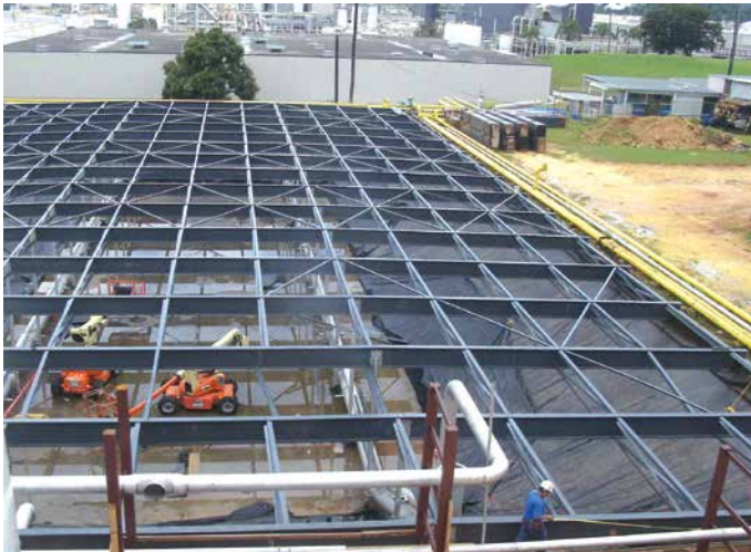
An odor control cover was constructed using EXTREN® structural shapes for a waste water treatment facility in Puerto Rico.
