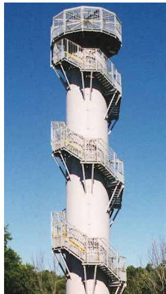
A system of FRP spiral stairs and landings supported by EXTREN® beams circle the Cordova Park Observation Tower at Red Rock Lake near Des Moines, Iowa.
