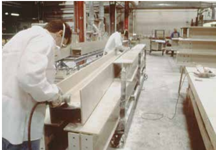
Beams are prepped before bonding connections together.
