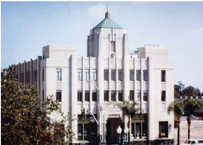
EXTREN® was used as trim on this Oakwood Commons building in Michigan because the beams have the aesthetics of steel, however, EXTREN® does not need to be annually repainted because of its corrosion resistance.
