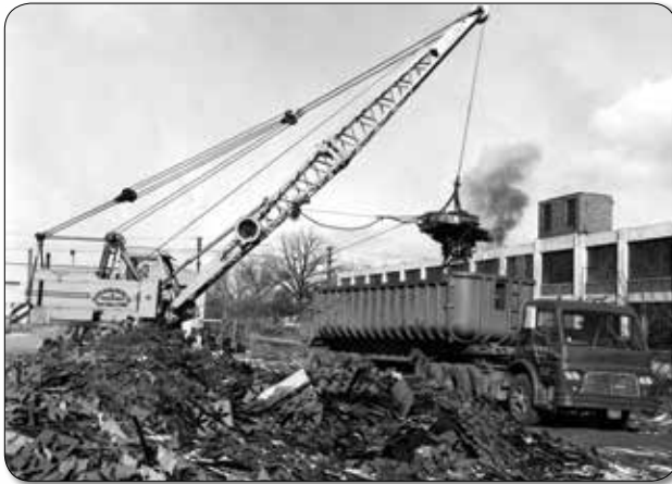
Glick Iron & Metal scrap yard - 1970s
