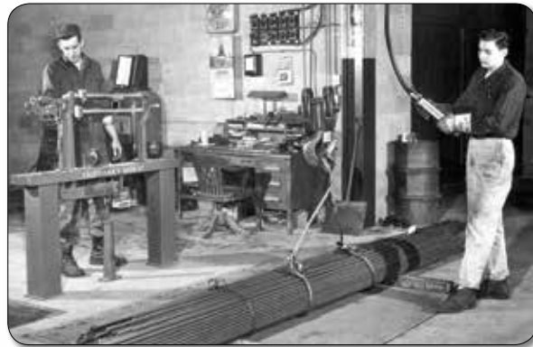
Roy Sprague at scales and Bill Horsh operating crane - 1952
