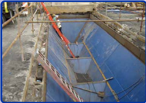
Four outlet phosphate receiving hopper lined with TIVAR® 88-2
