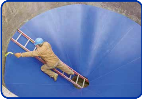
Some conical hoppers can even be lined with a one piece TIVAR® 88-2 "drop in" liner for a fast, clean installation
