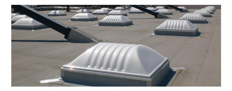
"Daylighting" is the use of "smart skylights" to distribute natural sunlight into a single story building and significantly reduce the need for electrical lighting. In response to a market demand to improve "daylighting", Covestro has engineered the TUFFAK SK polycarbonate sheet family of products to meet the varied but strict design requirements of "smart skylights".
