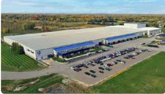
Pictured, the Alro Steel facility in Pottsville, Michigan
